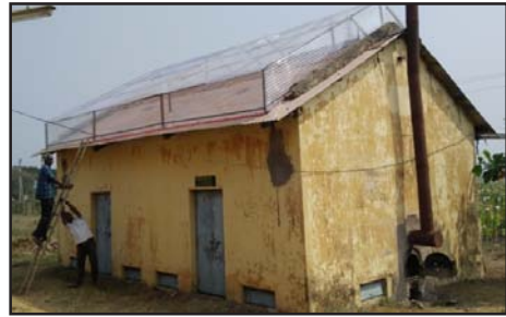
Fig.3: Polycarbonate roof barn designed and used for testing
